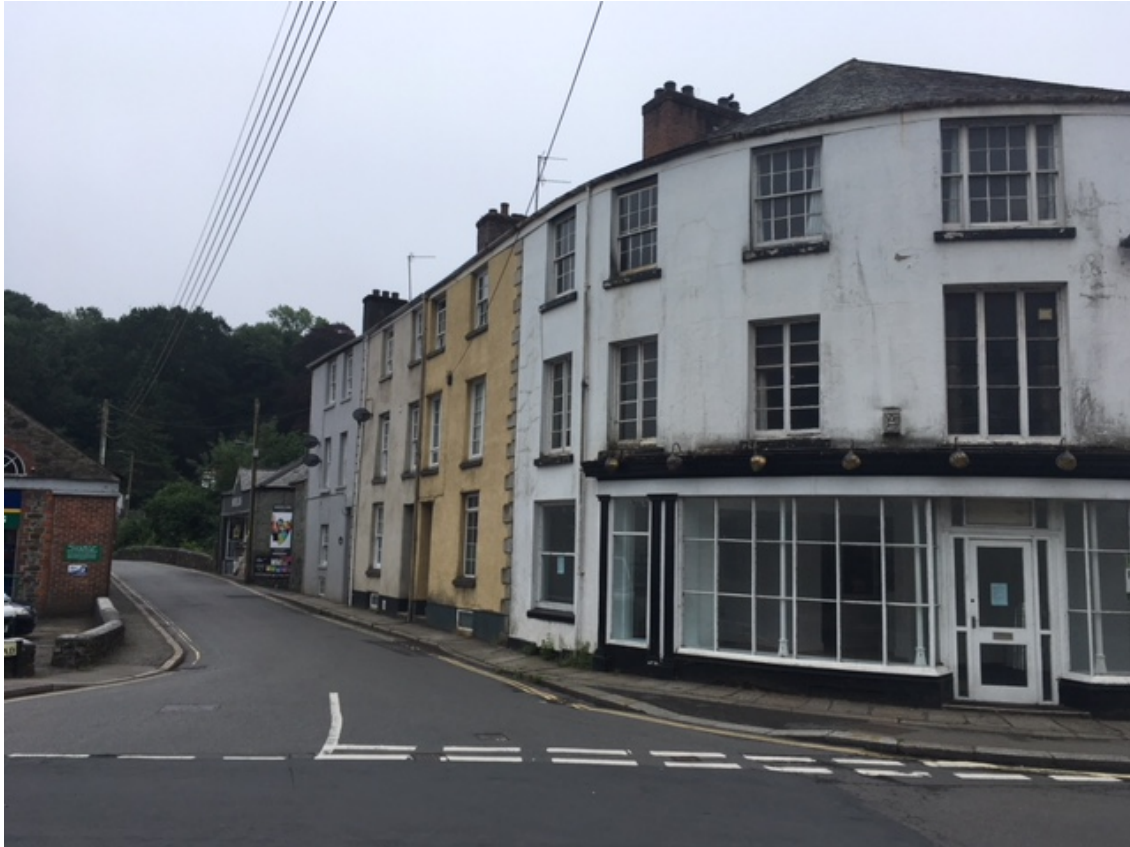
View south east along Vigo Bridge Road
